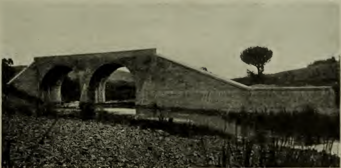
FIG. 4.—HAMMERSDALE SPRUIT BRIDGE.
